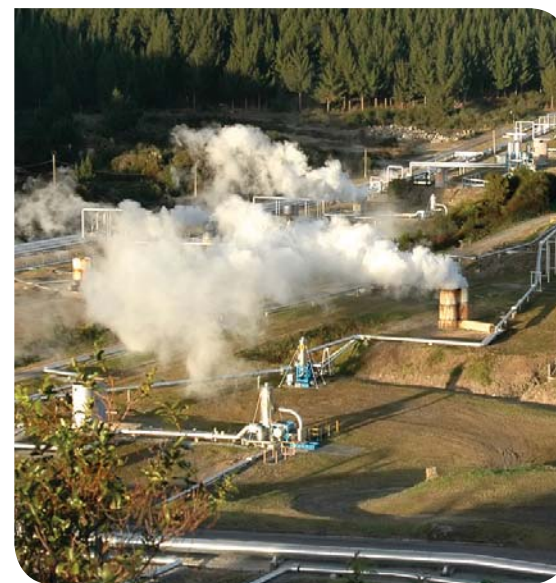
▲ In New Zealand, boreholes are drilled into the ground to collect the steam
